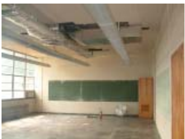
Almost cleared Computer Room New duct work overhead
