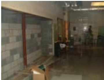
Old opening for new lockers
