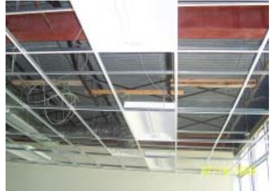
New ceiling grids, lights and wiring
