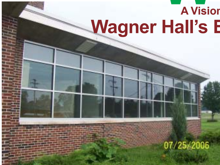
New energy efficient windows are installed
