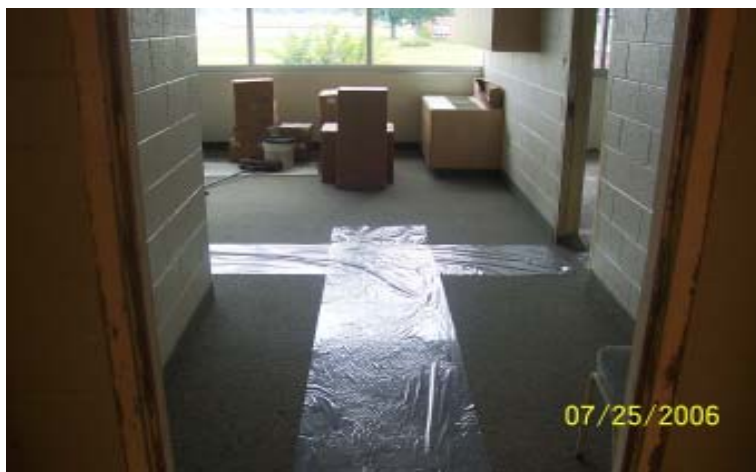
New carpet is installed in administrative offices
