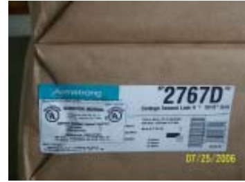
New materials on site
