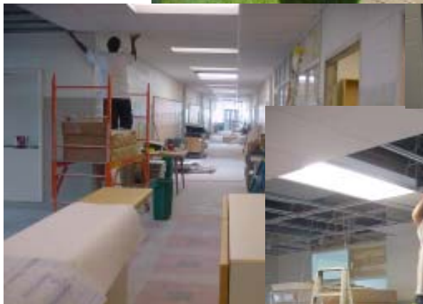
Ceiling tiles are installed down the hallway (above), in the classrooms, lobby (right) and library (below)
